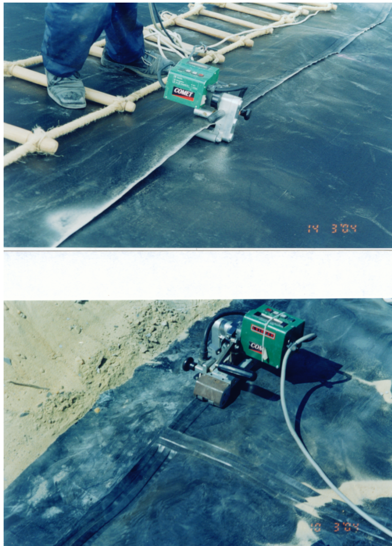
Welding with Hot Wedge Fusion Machine
