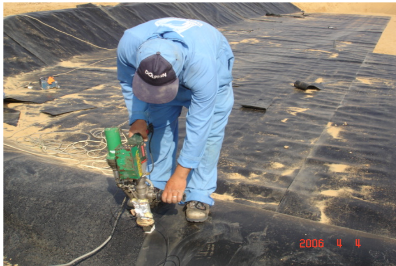
Welding with Extrusion Welding Machine
